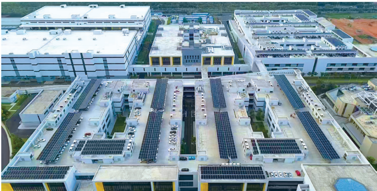
Photovoltaic Power Generation at Nanning Li Ning Center
