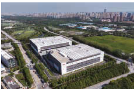
Appearance of Shanghai Jiading Logistics Park
